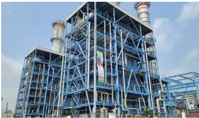
Bhola 225 MW Combined Cycle Power Plant
